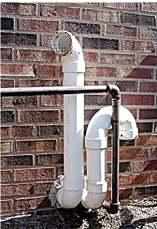
Outside Termination of Direct-Vent Pipe. (Courtesy of Magic Sweep Corporation)
