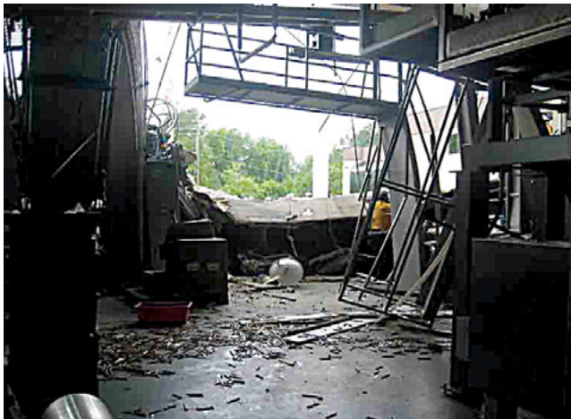
Interior of the ConAgra Plant after the Explosion.
