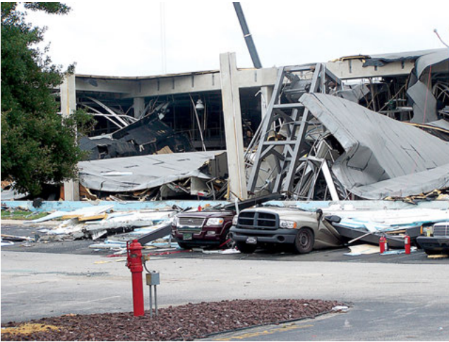
View of the ConAgra Plant after the Explosion.
