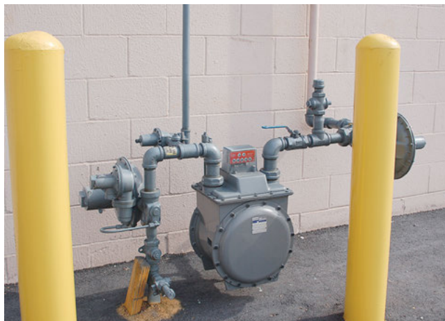
Gas Meter Protection. (Courtesy of AGL Resources)
