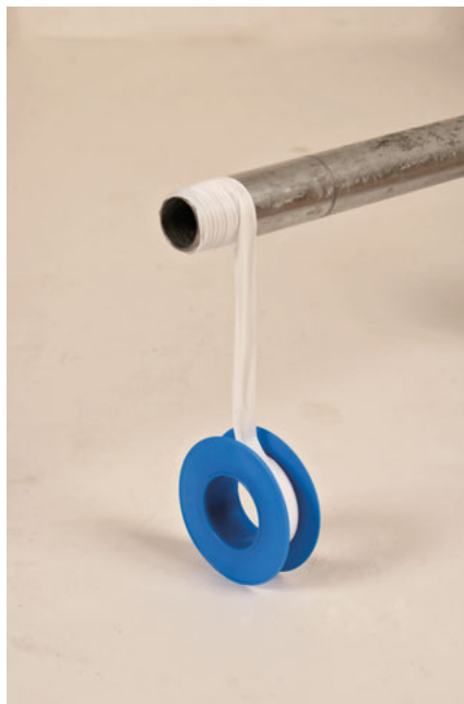
Winding PTFE Tape on a Male Pipe Connection. (Photograph by Krysta S. Doerfler, Fine Homebuilding Magazine © 2009, The Taunton Press, Inc.)
