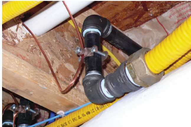
Bonding to Steel Pipe Near a Section of CSST, Using a Bonding Clamp.
