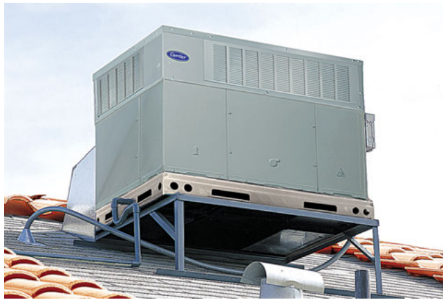
Example of an Appliance Roof Installation. (Courtesy of Carrier Corporation)
