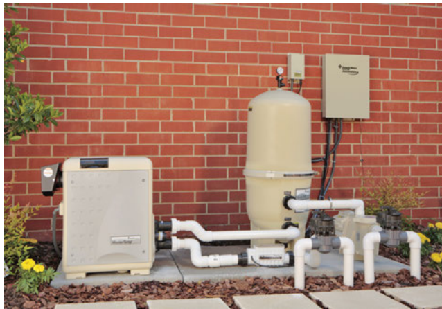
Pool Heater. (Courtesy of Pentair Aquatic Systems)
