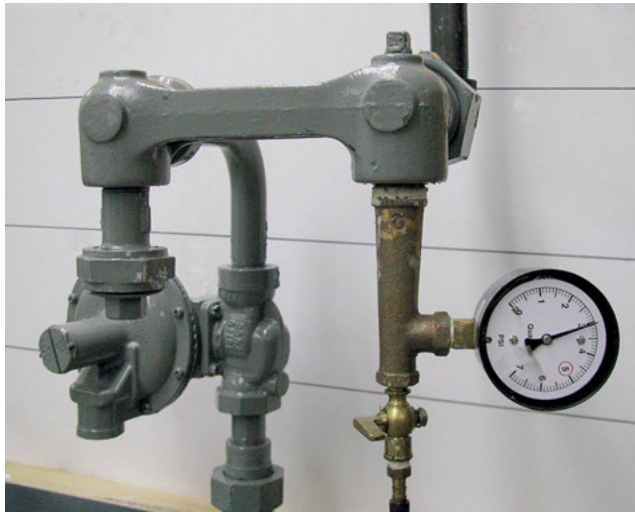
Pressure Gauge Installation. (Courtesy of NSTAR)
