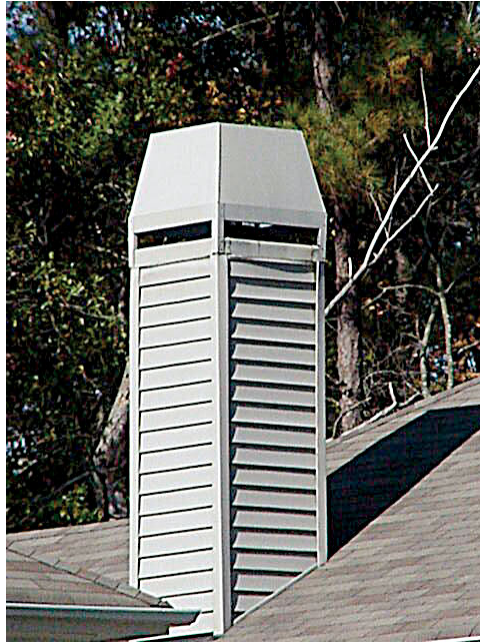
Decorative Vent Shroud. (Courtesy of Magic Sweep Corporation)
